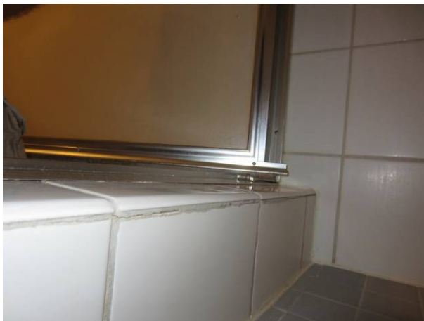
Cracked grout noted inside shower stall.
