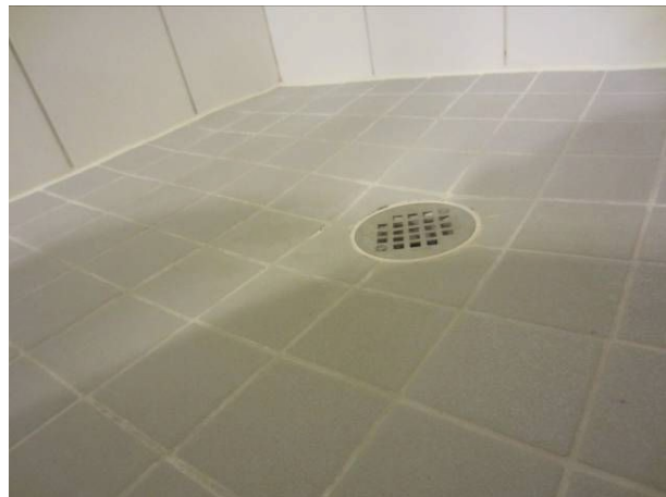
Cracked grout noted inside shower stall.
